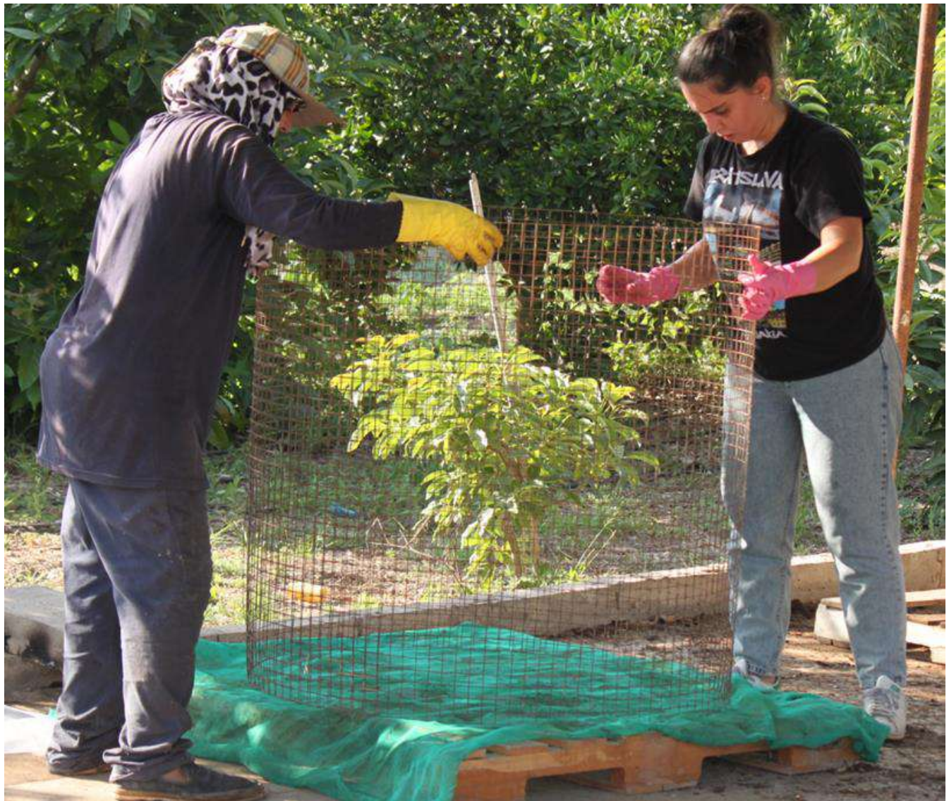
Compost pile structure construction (Photo courtesy of Nour Nahouli)
